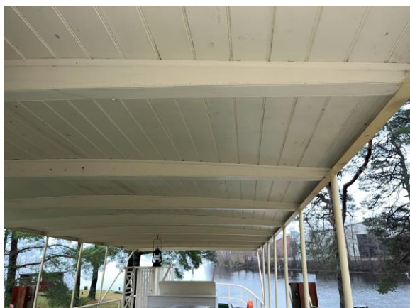
Himling, takoverbygning – dekk.
