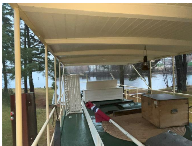
Himling, takoverbygning – dekk.
